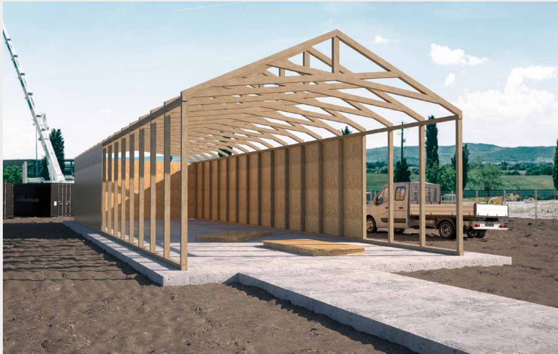
Fastening Wood Trusses outdoors.
